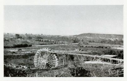
Before this wheel was built in the late fifties to raise water out of the Zanja, Los Angeles' domestic water was delivered from door to door in a cart
